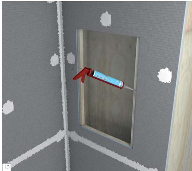
**EN** wedi Niches are installed in a cut out in the wedi wall and attached with its flange right into the center of 16 o.c. (406 mm) studs. wedi Joint Sealant is set along the connection of wall to niche.
