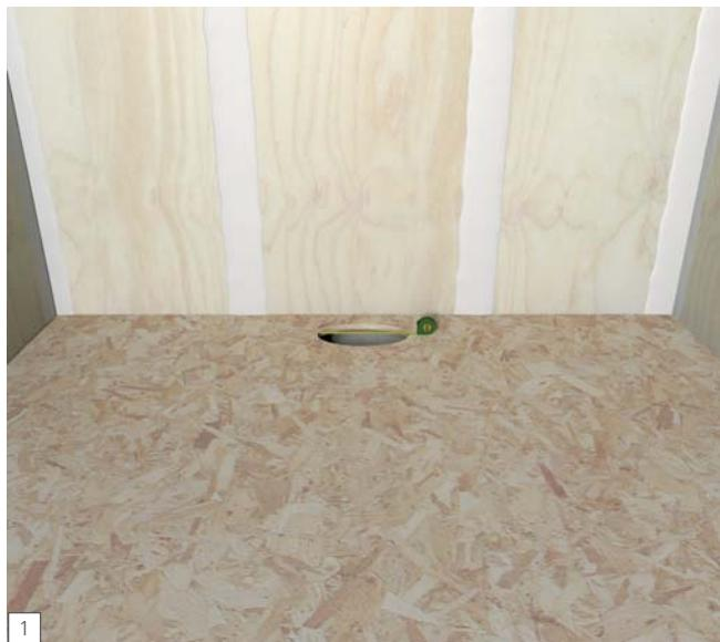
**EN** Cut the 2" pipe 1 1/4" below the top of the Subfloor. Use the oval shape cutting template where you want to position the drain to cut out subfloor using a jigsaw to allow wedi drain trap to be inserted and connected to floor pipe using appropriate ABS compatible or multipurpose cement glue. Please also check cement glue compatibility to floor pipe material. The drain and trap have to be secured to the subfloor. Drain recess cut out must not add deflection to subfloor.
