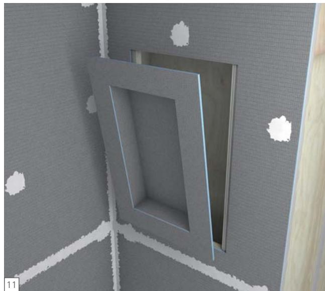
**EN** 2 Fasteners each side of the niche are set to create a flush transition to the wall panels. Another 1/2" bead of wedi sealant is spread over fasteners and seams.
