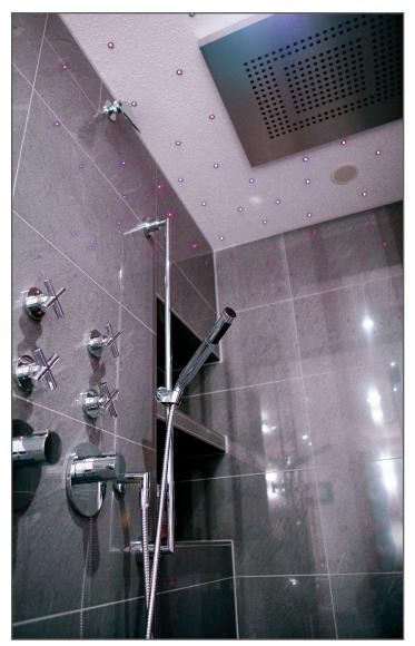
equipment and fixtures must be rated for submerged use and carry an IP 67 class rating. Lighting may produce heat and such heat should always be projected away from structures. Caution is necessary when working with lighting commonly used in pools. These are often cooled by the pool water which does not occur in steam rooms. All metal based equipment and fixtures should be corrosion resistant on the level of stainless steel 316.
