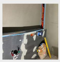
After the walls and floors were stripped, waste and fresh water pipes were re-routed. The bathtub got replaced with a flush-to-floor wedi Fundo Primo shower element creating a shower space that is safe to use for everyone. The floor was levelled off with wedi building boards to create level access to the shower as well as to waterproof the entire floor surface. In order to maximise the available space and create barrier-free access to the bathroom, the door was replaced by a large sliding door.
