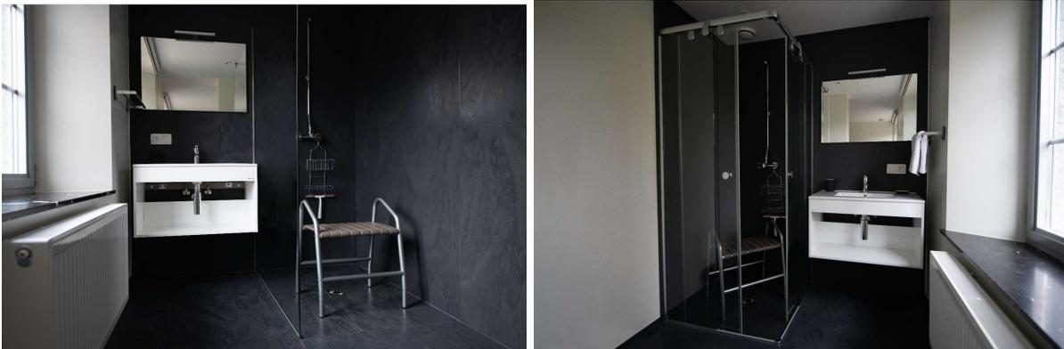
Despite the wooden floor, the flush-to-floor showers in the Sourmont Abbey could be implemented with wedi elements. The built-in shower element and the walls were then covered with the carbon black design surfaces of the wedi Top Line.
