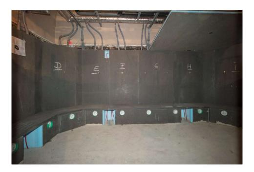
The walls in the laconium and steam bath areas of the Neptunbad consist of prefabricated wall elements, which the processor only had to set up and bond together. The benches were also prefabricated at the factory. A test set-up in the wedi factory hall ensured that all elements fit perfectly on the construction site.
