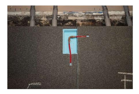
Optimally coordinated works steps ensured the fast project completion at Nebtunbad: after the arrival of the prefabricated wall elements to the construction site, the walls were simply bonded together and the pipes got connected by the installer.
