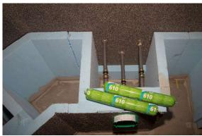
I-Boxes and connection pipes for the carrier elements of the benches were already installed and sealed at the factory. Before seat surfaces could be bonded to the carrier elements with wedi 610, the pipes were connected by the installer.
