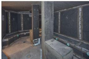
Wolfgang Peters built the columns to the ceiling for the steam outlet with the steam box on site from building boards. Special mounting plates were glued in the columns, into which the installer could attach the steam, condensate and air supply lines for the steam box.
