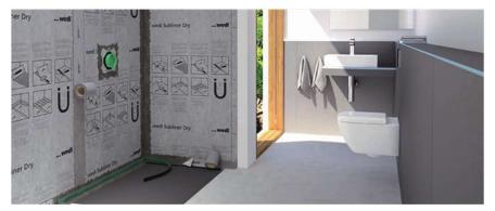
Whichever design solution is chosen, floor-level showers must always be permanently waterproof themselves as well as securely connected to the wet room's tanking system. In principle, it makes sense that all components are coordinated with each other, and have also been tested and approved by building authorities.
