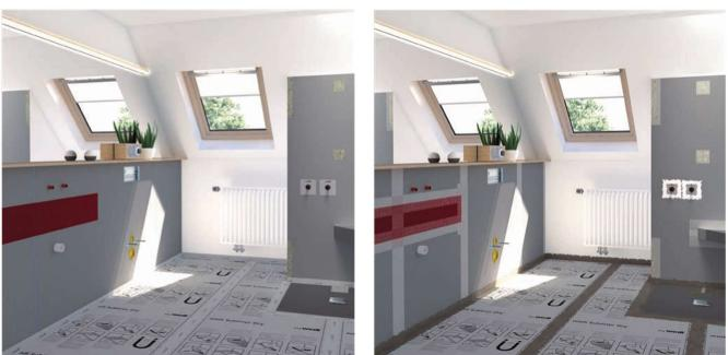
Drain technology, sound insulation, fire protection - many aspects have to be considered when planning floor-level showers properly. The existing floor structure i.e. the maximum available construction height and the slope – is a key factor for the design.
