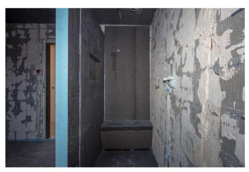
The shower was separated from the rest of the bathroom by the practical wedi Sanwell wall element, providing the necessary intimacy while at the same time adequately protecting the walking area from splashing water.
