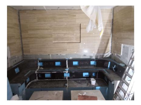
Due to the high degree of prefabrication of wedi elements, technology systems simply just needed to be inserted into the pre-milled cavities on site.
