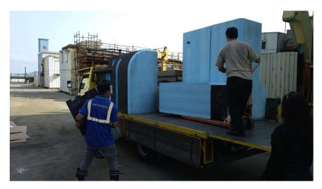
All individual components were delivered to the construction site in finished form. Thanks to them being lightweight, even the large parts were easily carried by one person.
