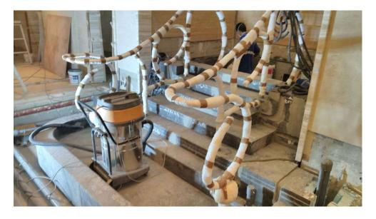
As the elaborate set of handrails fitted on the steps were very heavy, individual wedi elements were reinforced to be able to carry their weight and the handrails were also secured to the floor.
